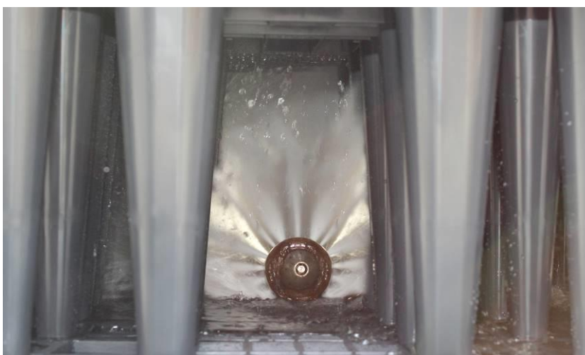
The EcoBloc Inspect Smart can be cleaned by high pressure jetting
